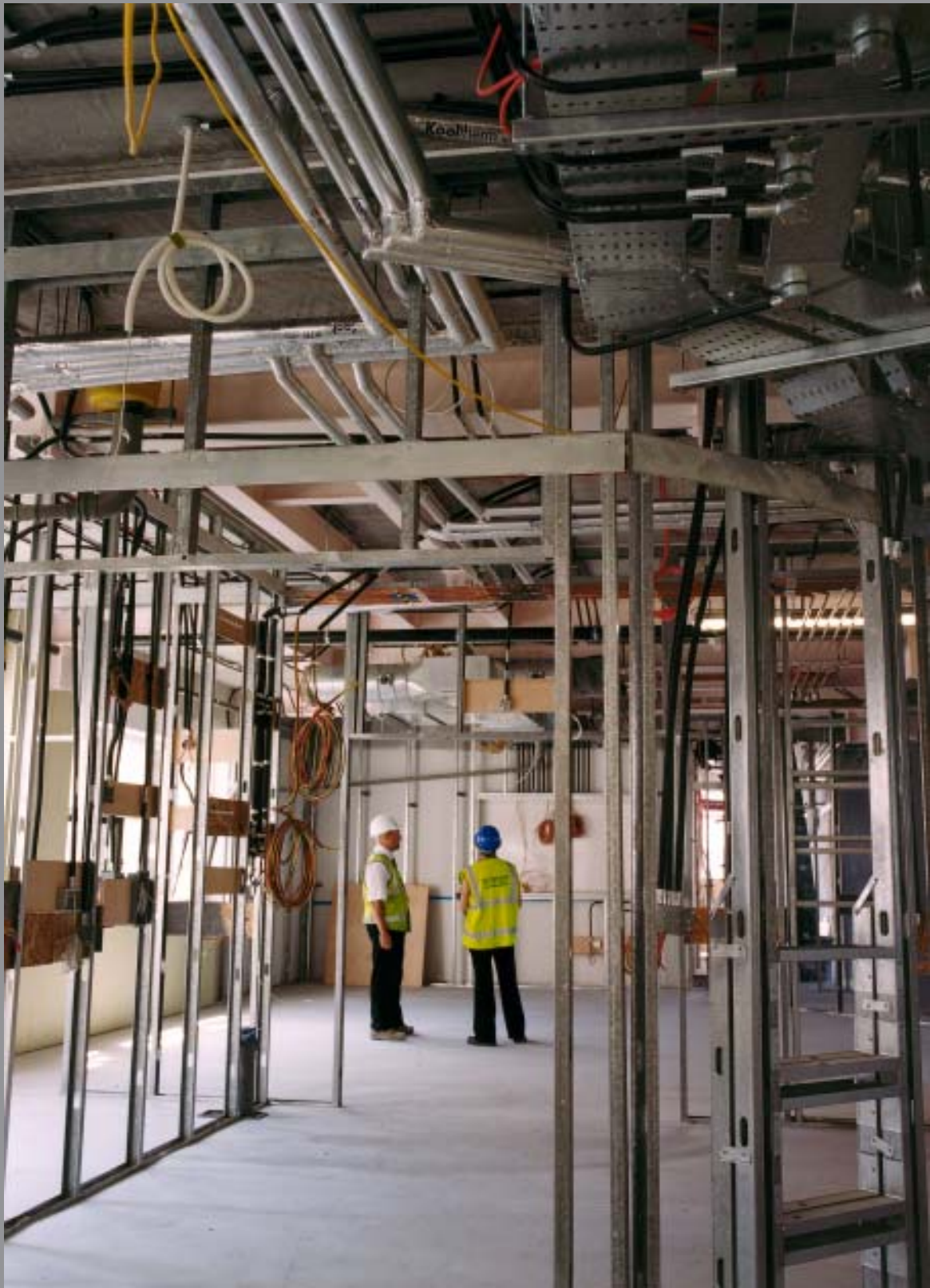
The interior works at the new hospital in Europort
